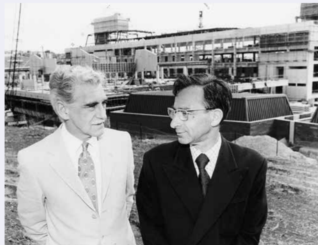
Professor Gus Fraenkel (right) at Flinders Medical Centre construction site with FMC administrator, Norman Popplewell, 1973.
